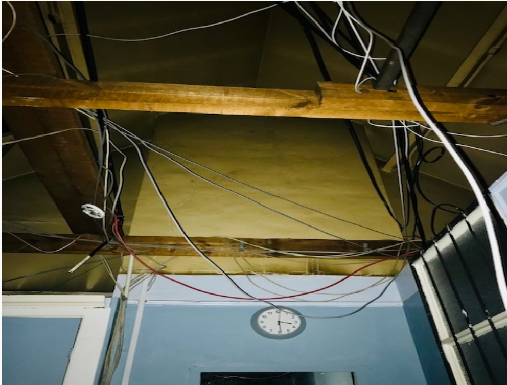
Lower Hall caretaker's space along with a plethora of old and new service cable and old metal conduit for old lighting.
