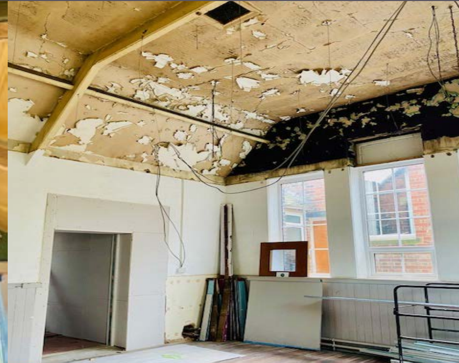
Room A suspended ceiling removed original ceiling exposed and plaster issues revealed
