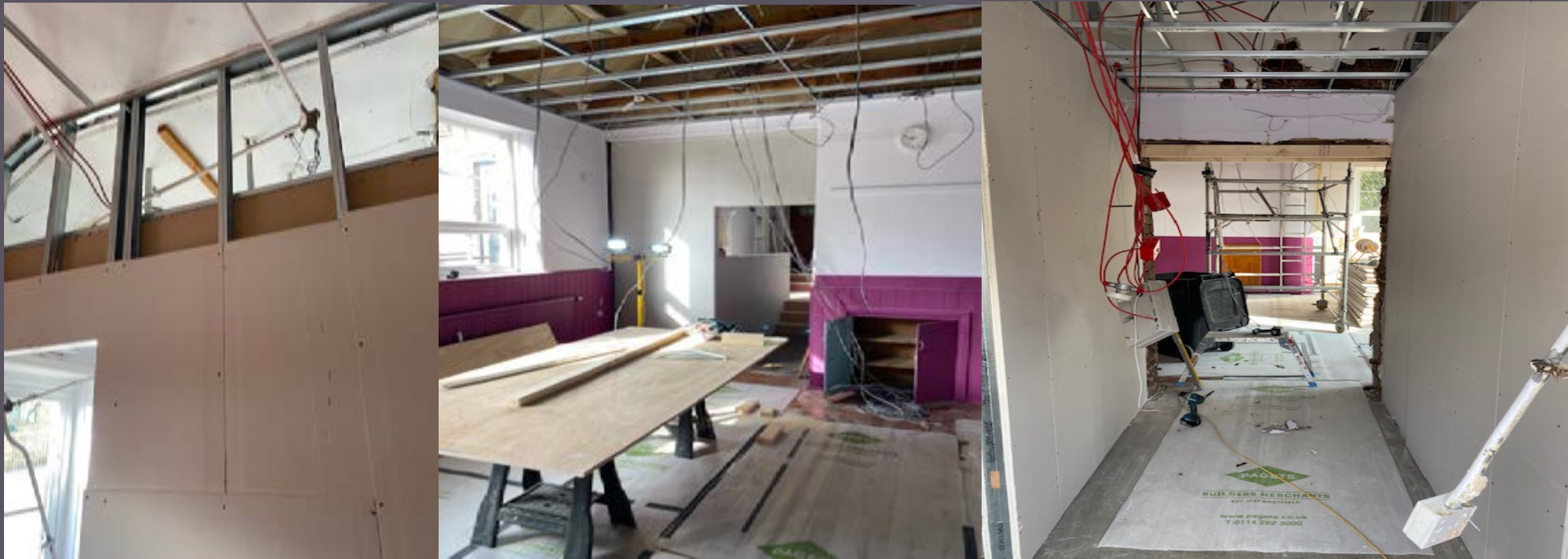
New stud walls lower hall and framework for new ceiling in the lower hall.
