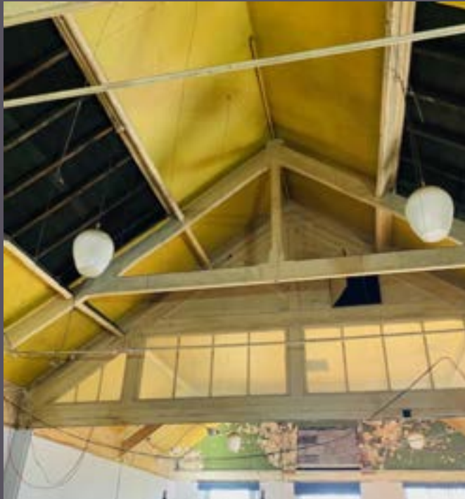
Upper Hall suspended ceiling removed exposing old roof and roof lights, beams and partition walls with original glass and 1950s hanging light.
