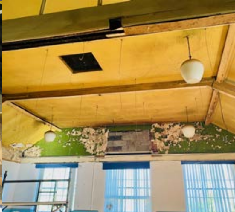
Upper Hall suspended ceiling removed exposing old roof and roof lights, beams and partition walls with original glass and 1950s hanging light.
